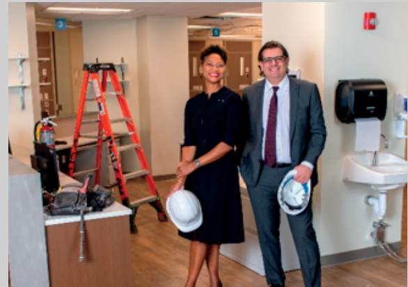
Photo: Stacy Anne Mehciz, MPA, BSN, RN and Emre Kayaalp, MD, PhD check out the maternity center renovations currently underway.
